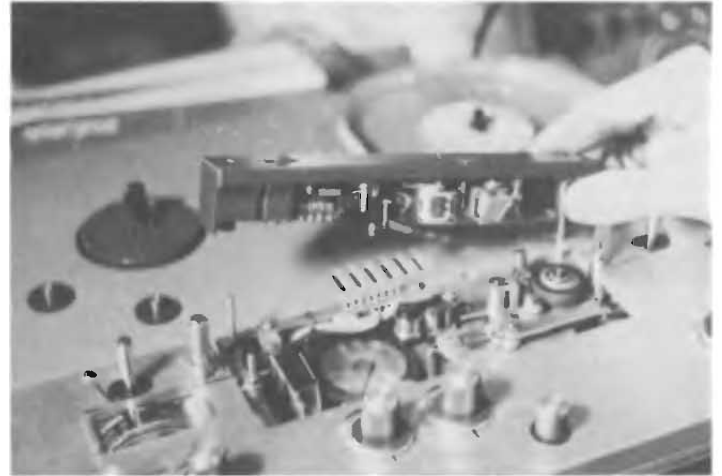
Fig. 8 —The Ultimate! In this Uher Varicord design, the complete head assembly can be removed and interchanged for different track formation. Accurate machining of mountings is the secret.
