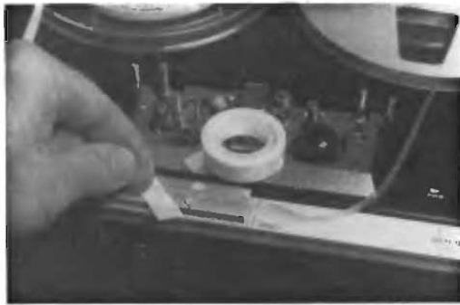
FIG. 6—INITIAL BURNISHING IN THE BLOCK
